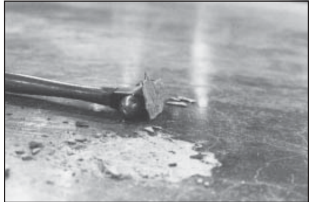
Delaminated Concrete
