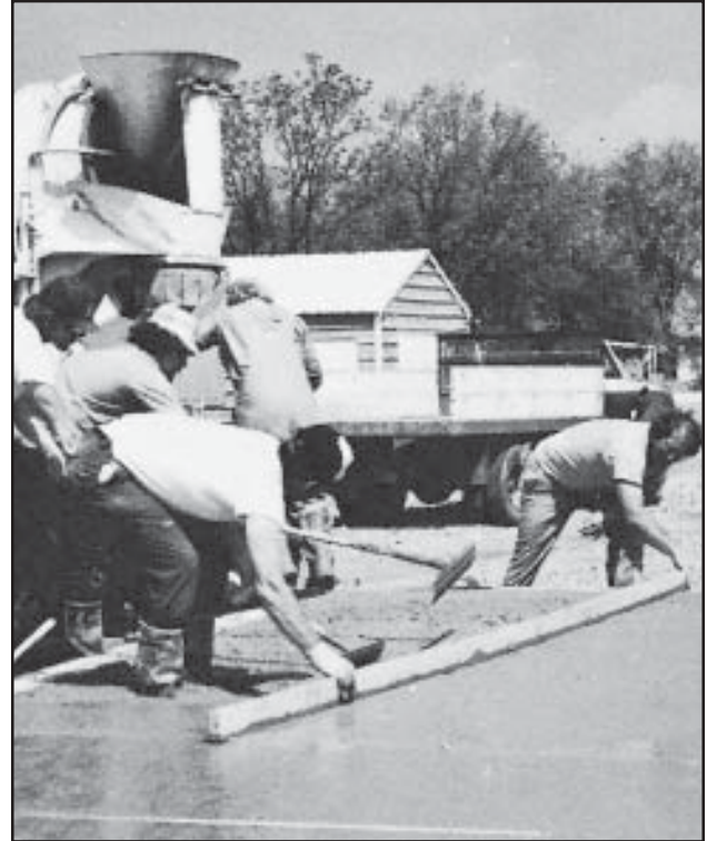
Finishing Concrete Flatwork
